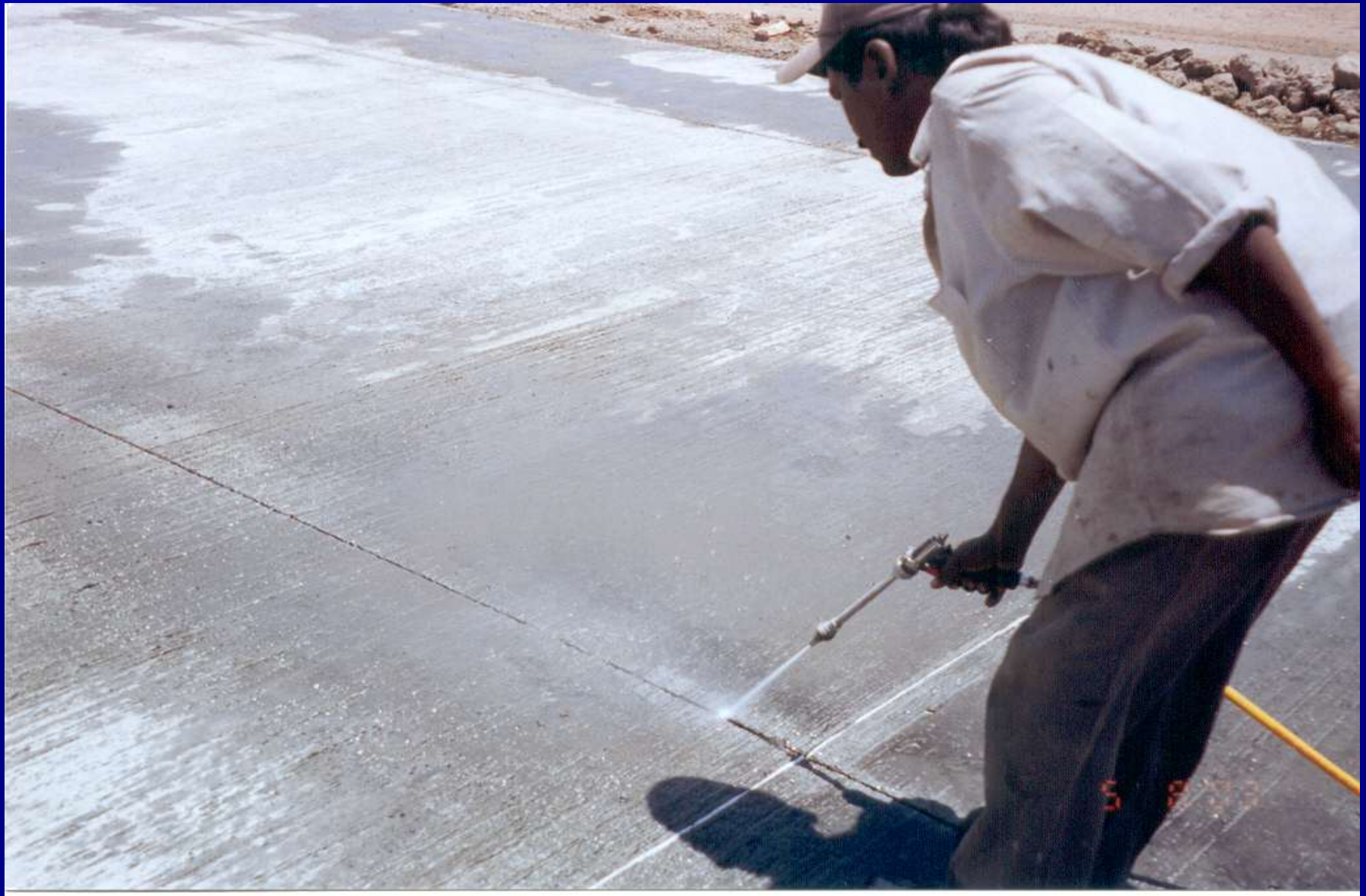
Cleaning of Longitudinal Joint
