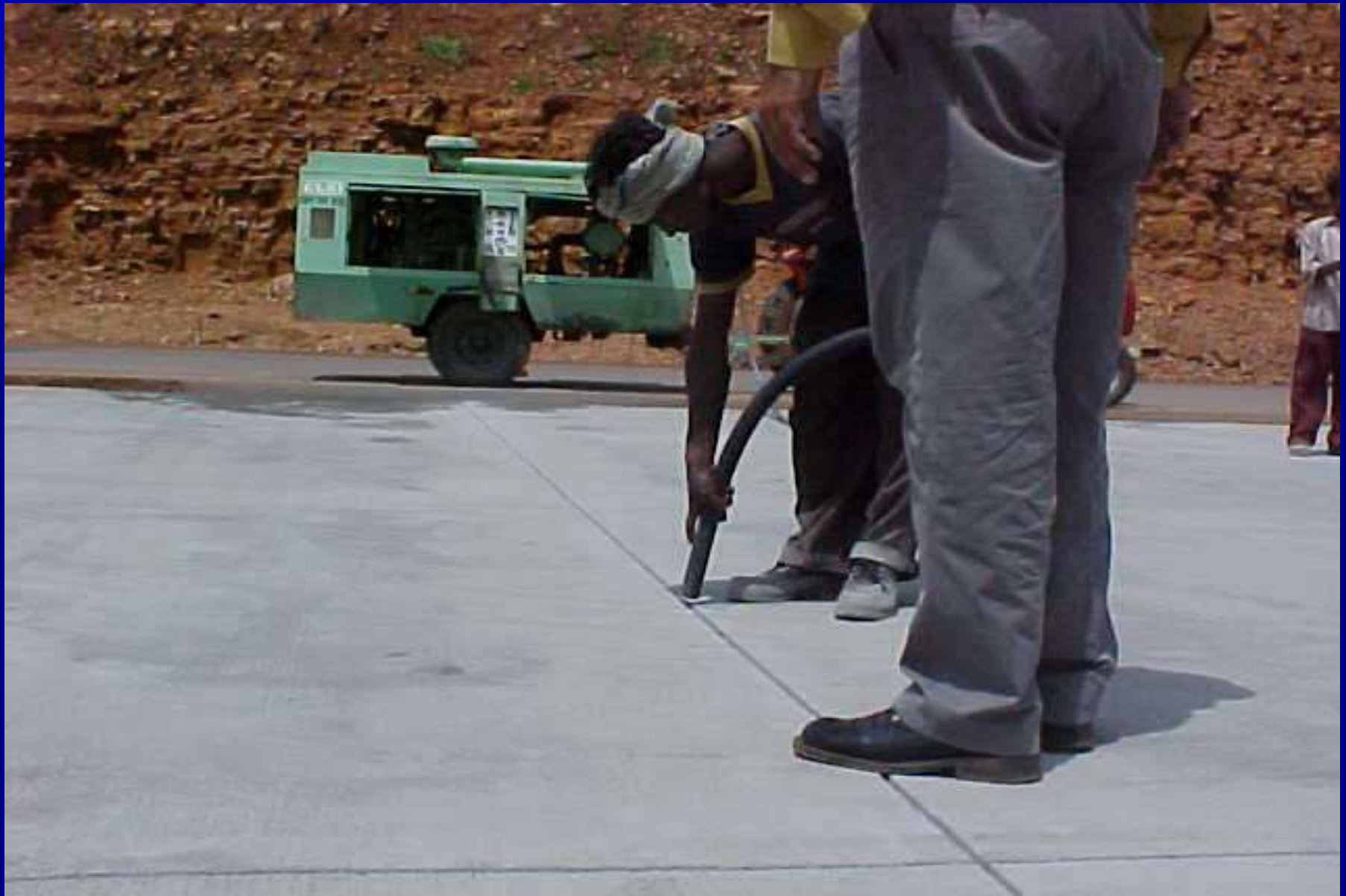
Cleaning of Groove with Compressed Air
