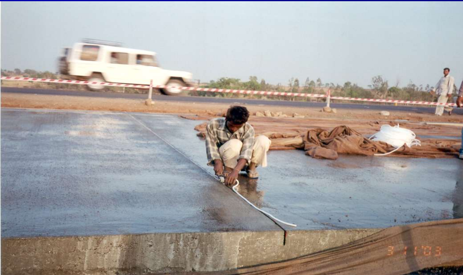
Fixing of Back up Rod after Initial Cut
