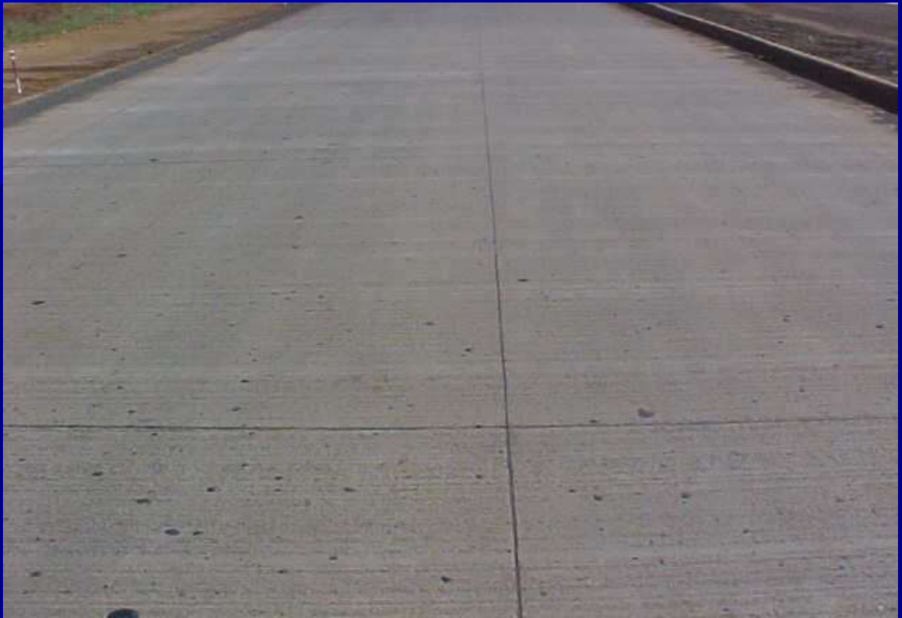
Finished PQC surface with Sealed Joints
